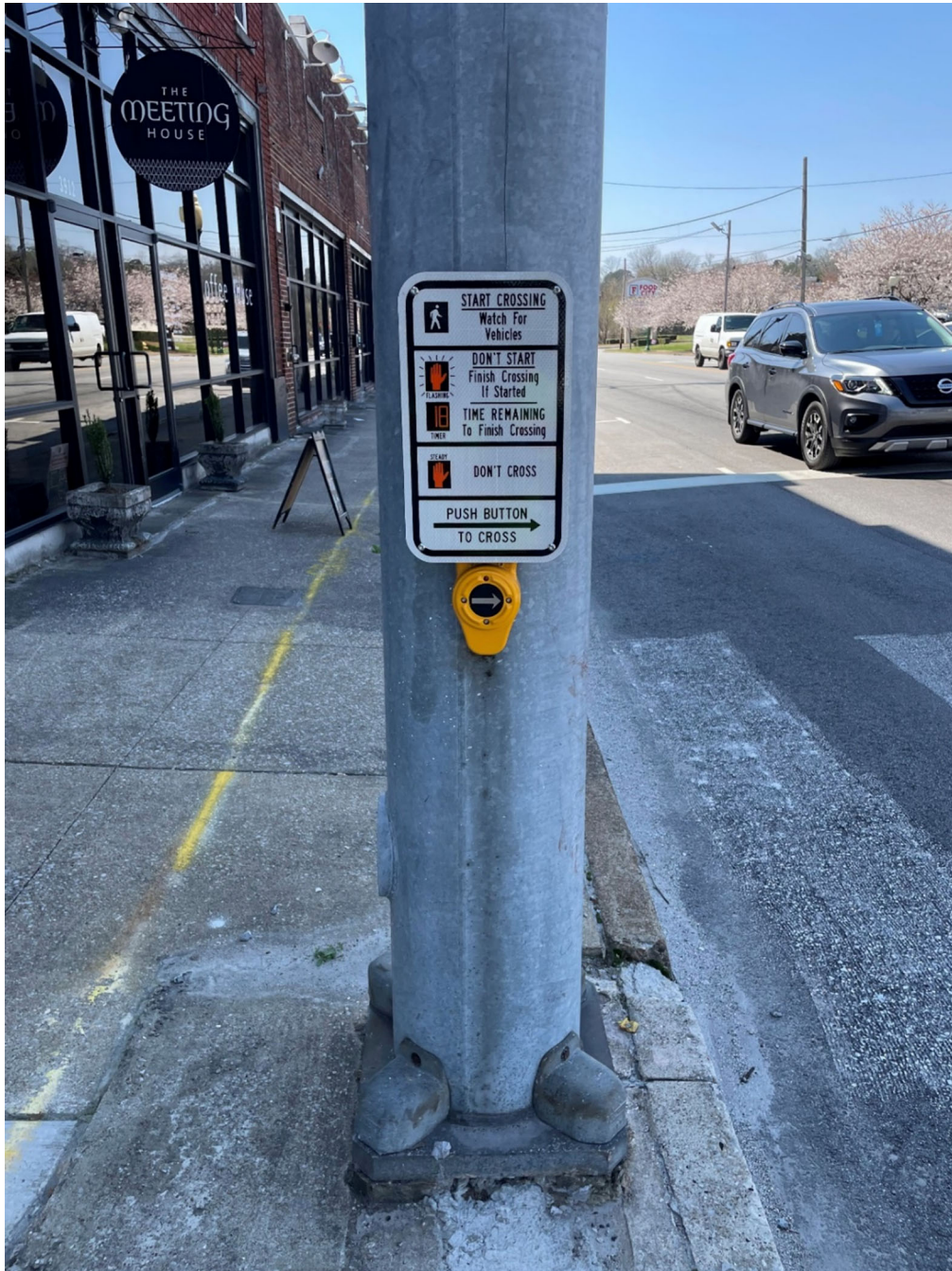
Figure 9 – Southeast Corner Pushbutton for crossing Dayton Boulevard
