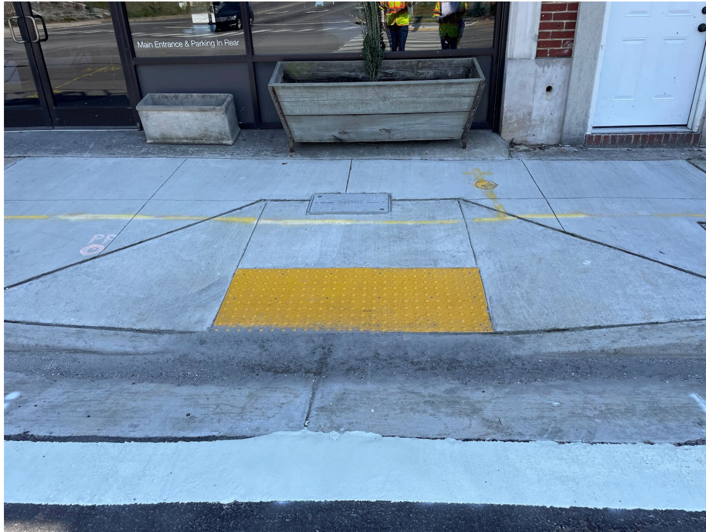
Figure 18 – Southeast Corner Curb Ramp
