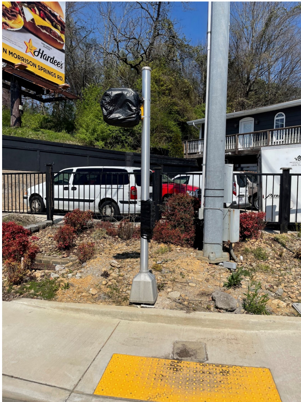
Figure 8 - Northwest Corner New Pedestrian Signal Head with Pushbutton at channelized crossing
