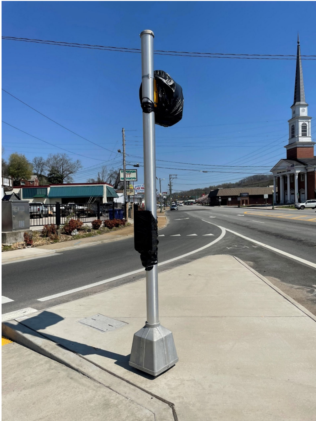
Figure 6 – Northwest Corner New Pedestrian Signal Head with Pushbutton on Channelization Island
